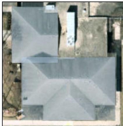
South & West Portion Administrative Offices & Police Department
